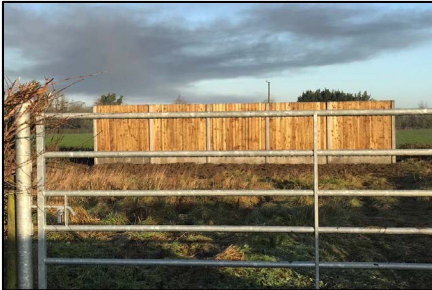
Hoarding on NPR
