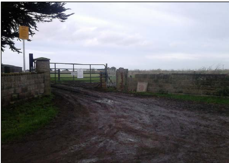
Proposed repair of pillar and wall at Sandyhills
