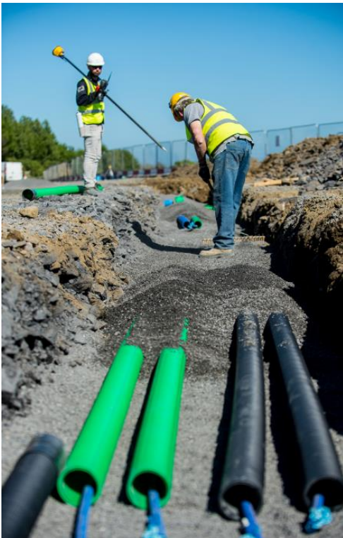
Installation of Utilities
