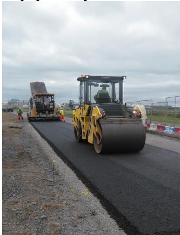
Realigning and building new Roads
