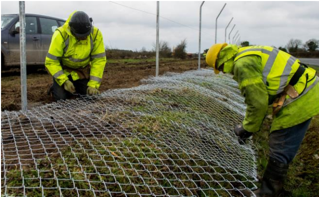
Installation of Fencing
