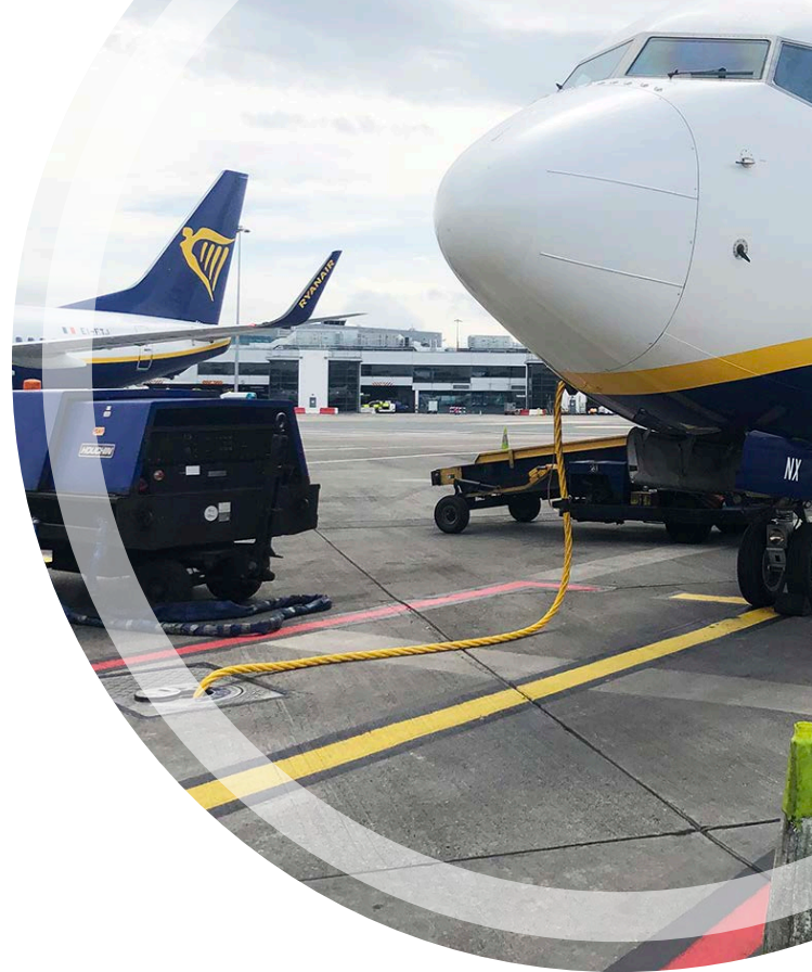
Fixed Electrical Ground Power (FEGP)
